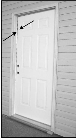
*In the above pictures, the weather-stripping is not evenly compressed from top to bottom, which may cause air and water infiltration and, therefore, frost during cold weather.*
