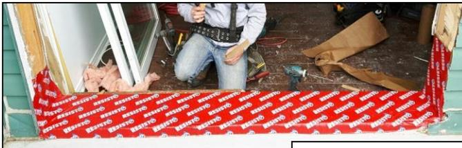
Flashing with auto-adhesive membrane (across and up the lower part of the jambs).
